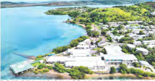
The affordability of building homes in the Torres Strait, in places like Thursday Island, is a major issue, says TCICA chief executive Mick Miller. Picture: Brendan Radde
